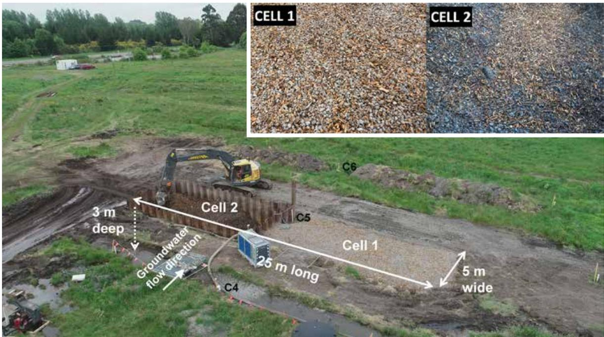
**Fig. 14.** / Pictures of the 50/50 woodchip/gravel mixtures that make up the denitrification wall, and a showing installation works. Cell 1: chipped wood mixed with 20-40mm gravel rounds. Cell 2 hogged wood mixed with parent aquifer material, screened of material under 20mm diameter. The positions of monitoring wells C4:C6 are marked on the photo.
